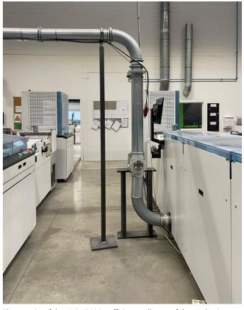
The capacity of the HKS-4500 is sufficient to dispose of the production waste on two finshing lines.
